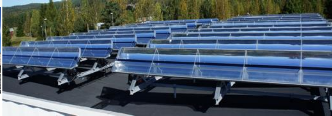
Parabolic Collector Quelle: Industrial Solar
